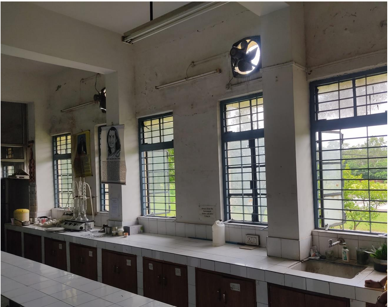
Figure 3 Wider and bigger Windows to allow natural light into the building
