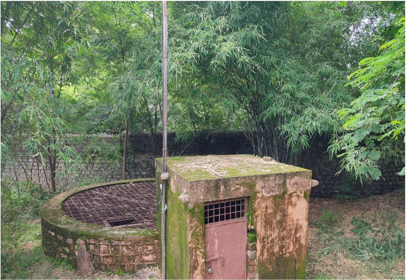
Figure 15 Rain water recharge well
