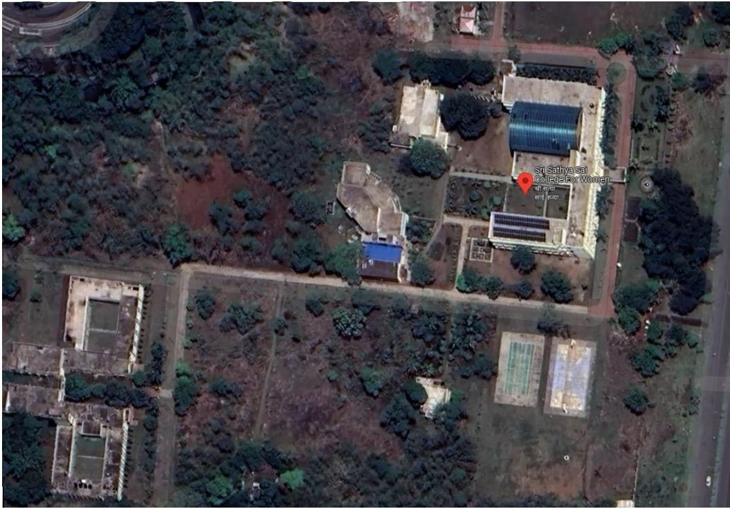
Figure 1 - The infrastructure aerial view of the campus
